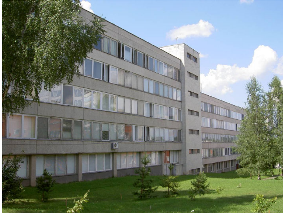
Fig. 1. Laboratory Building of Vilnius Gediminas Technical University (VGTU) before renovation
