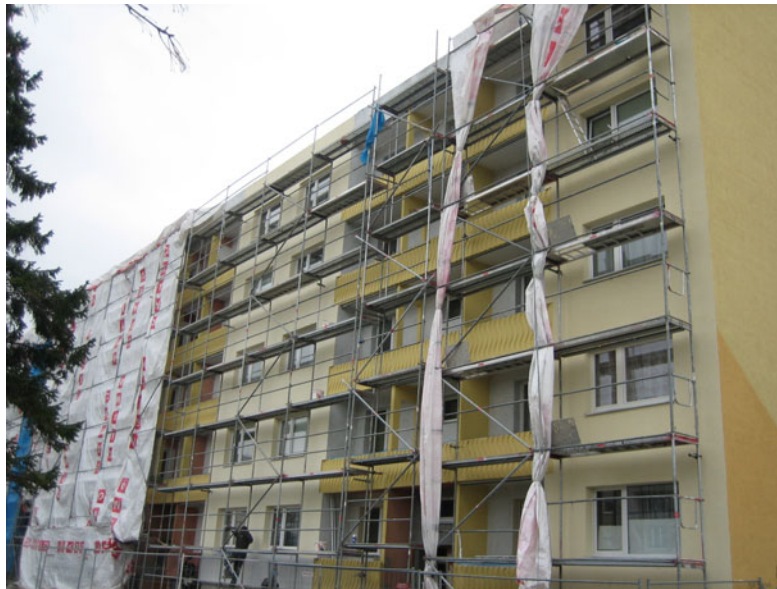
Figure 3: Balconies under construction.
