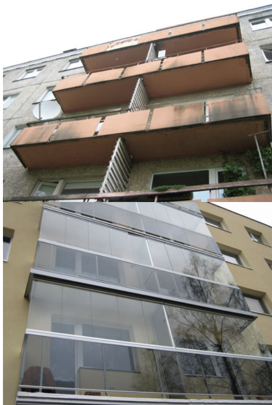
Figure 4: Balconies before renovation and after.
