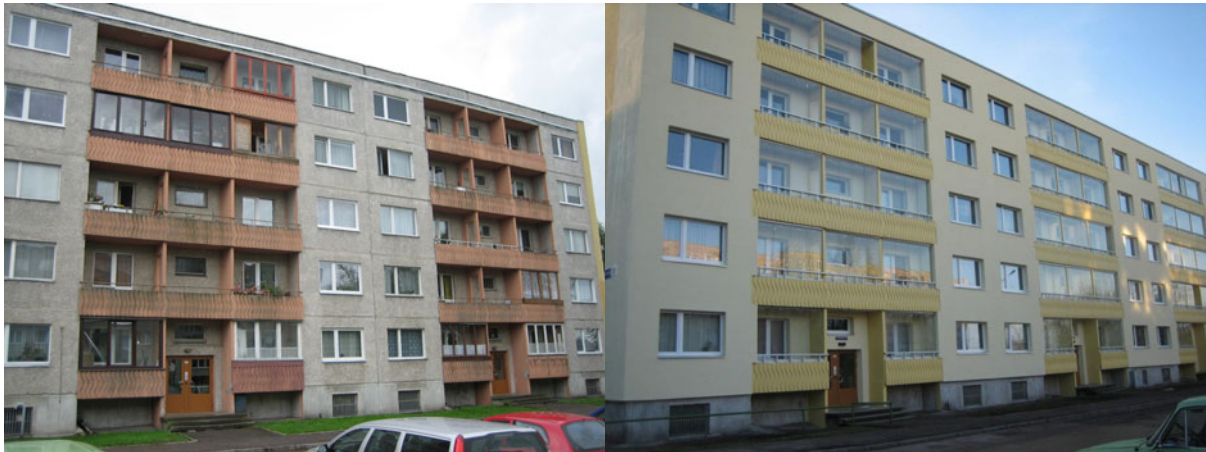
Figure 2: Façade of the apartment block pre and after reconstruction
