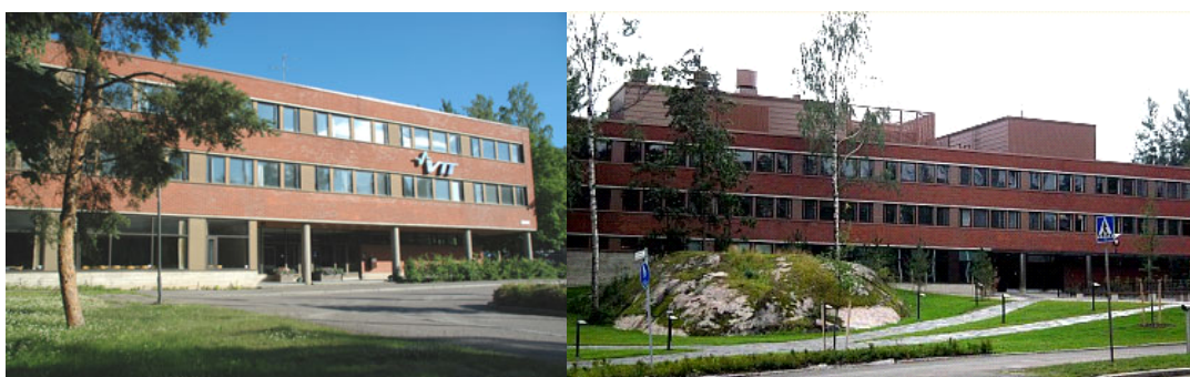
Figure 2: VTT office building before (2005) and after (2007) renovation.
